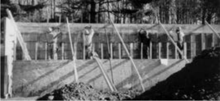
Miller & Long staff building grandstand walls in February 1999.
